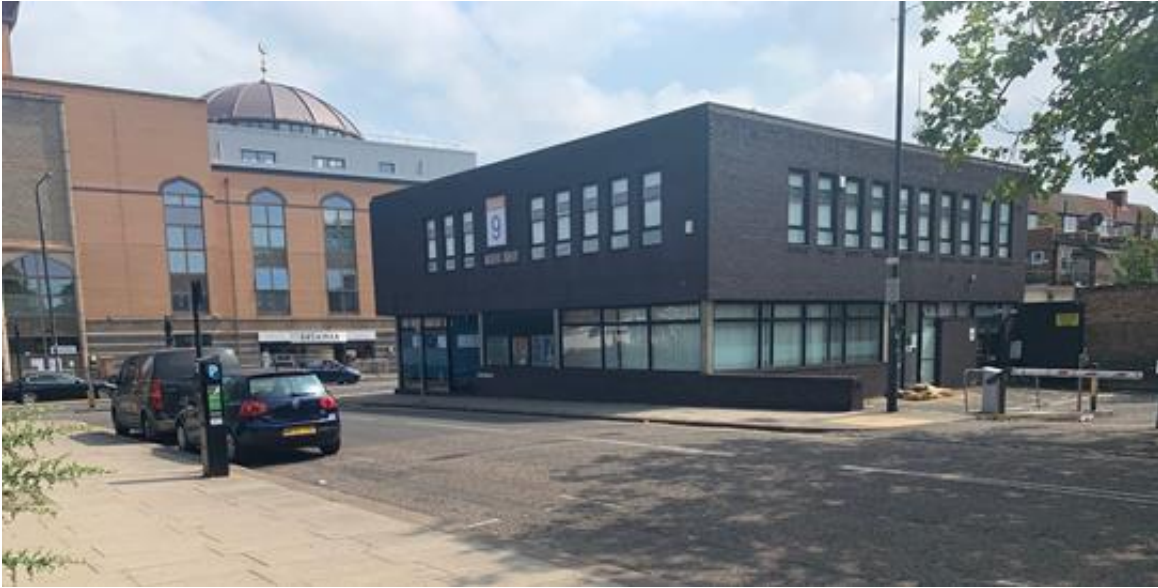
Side/Rear Elevation of Civic 9
